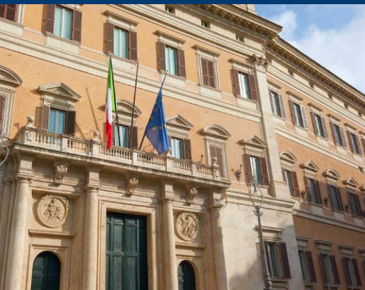
Main entrance of Palazzo Montecitorio, the seat of the Chamber of Deputies (the lower house of the Italian Parliament) in Rome, Italy.
